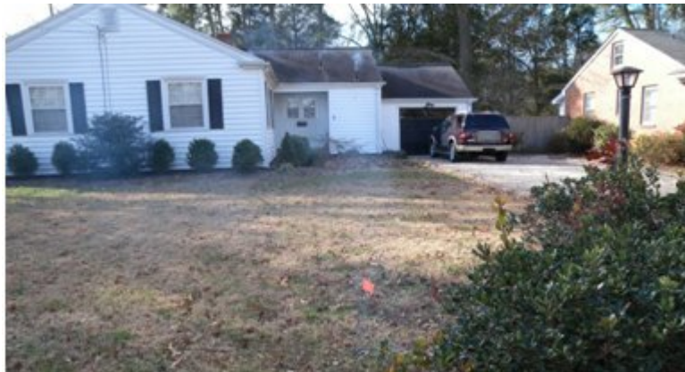
Smoke coming from vents in house roof
